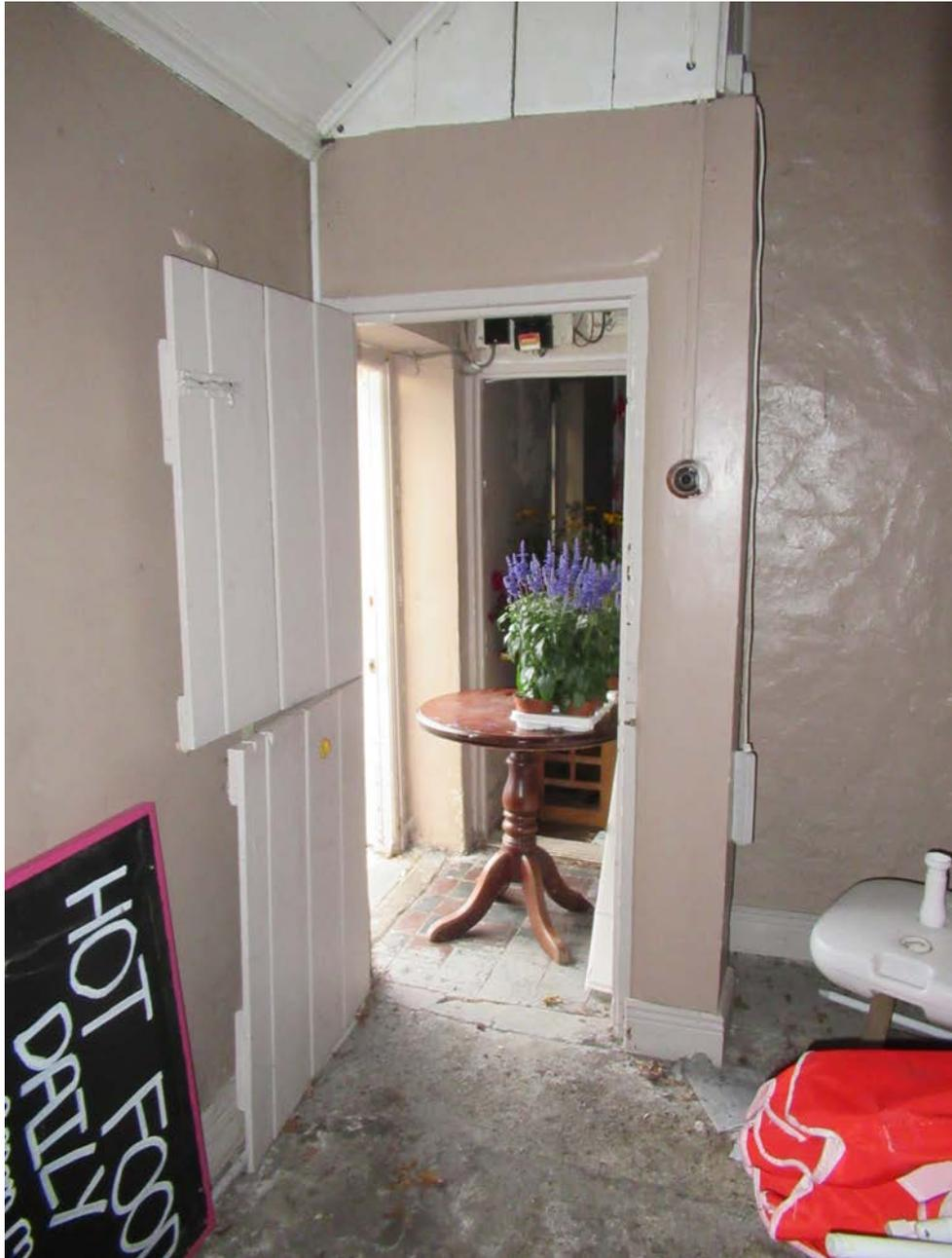
*Plate No. 10. Internal view looking towards the entry from the east room in the cottage. The entry is paved with red and black terra cotta tiles, commonly used during the late 19<sup>th</sup> and early 20<sup>th</sup> centuries.*
